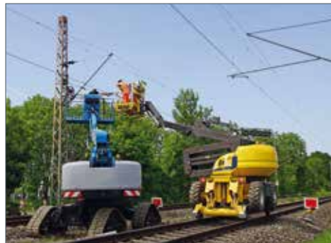
Construction of contact lines
