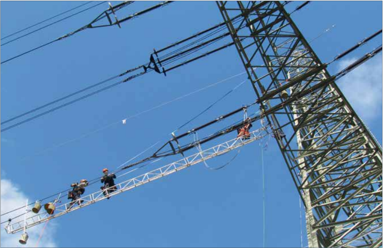
Overhead line construction
